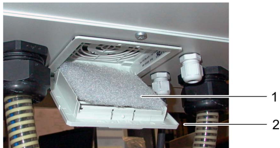
Fig. 5-8: Exchanging the lower filter mat
