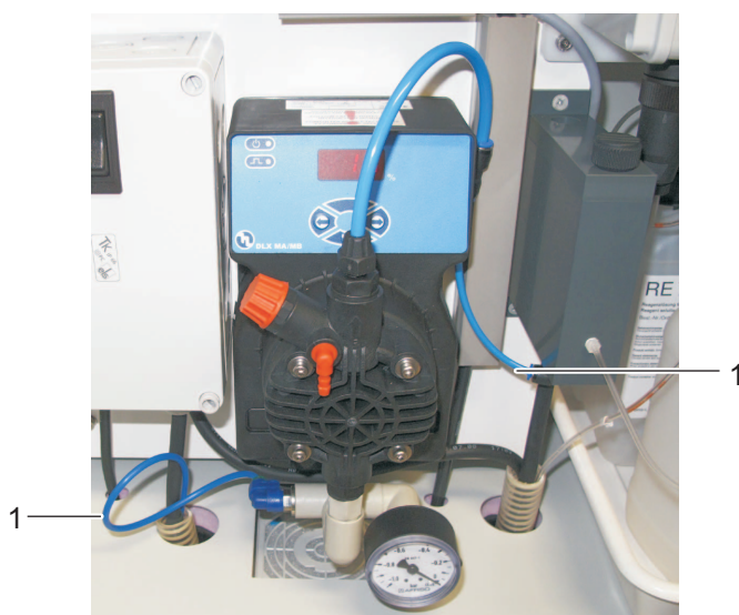
Fig. 5-23: Filtration pump with suction tube
